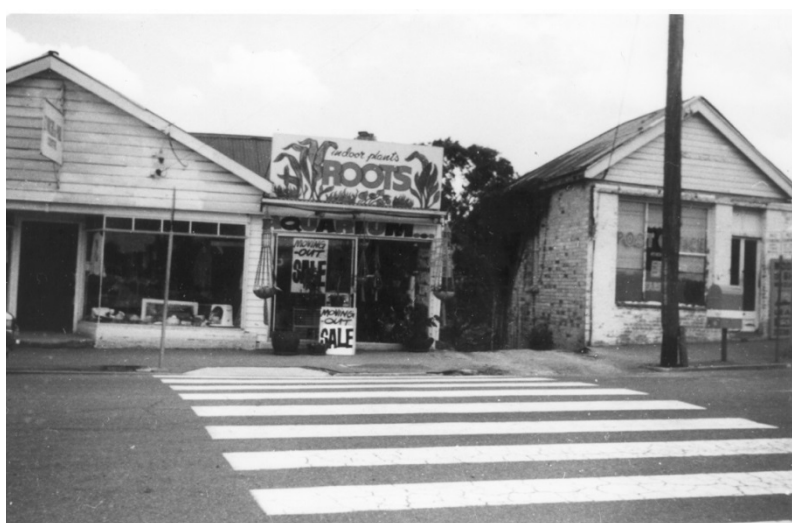
Taringa Post Office (right hand side of driveway) Moggill Road in the late 1960s/early 70s (Courtesy Judy Magub) - building already looks in a sorry state, by the end of the 1970s other photo's suggest the roof was about to collapse
