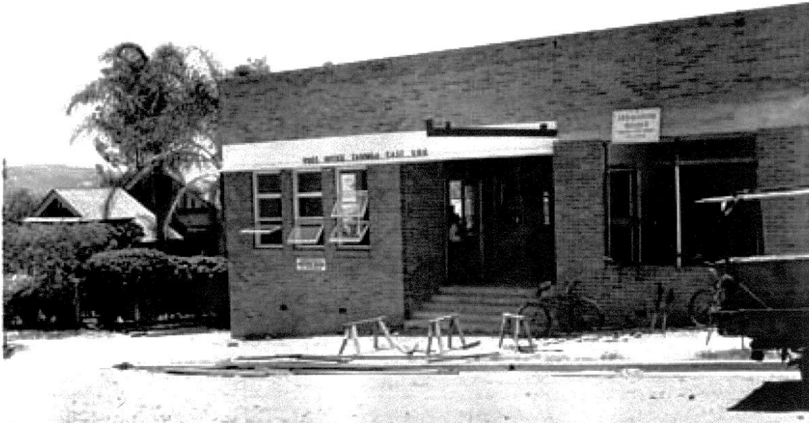
Taringa East Post Office nearing completion (National Archives)
