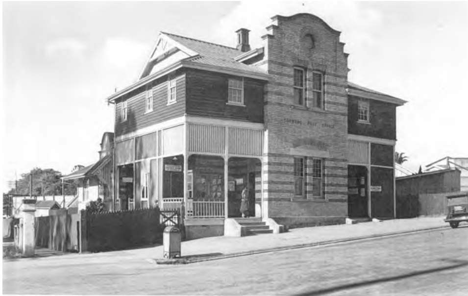
Toowong Post Office noted as around 1910 but possibly later (National Archives) – note original first floor verandah built in to provide more space perhaps when the upstairs area was converted from residential quarters to telephone exchange
