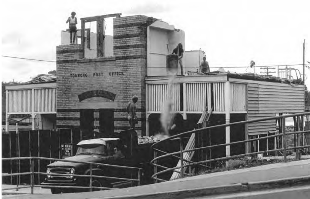
Demolition of the original Toowong Post Office early 1970s (National Archives)
