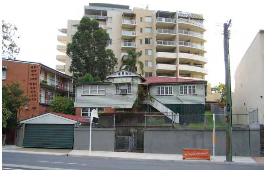
1930s Indooroopilly Police Station in 'Ferry Road' now Coonan Street (Author 2006)
