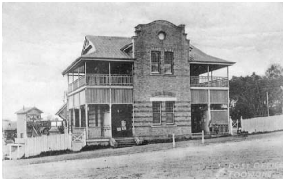
Toowong's first purpose built Post Office, post office services on the ground floor (front rooms), living accommodation on the upper floor (three bedrooms and a bathroom) and the rear single story wing (Dining Room, Kitchen, Pantry, Wash House and Servant's Room) – assumed all for Mrs Ferguson and her family. (National Archives)
