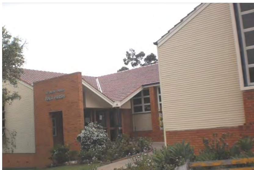
The entry between first and second churches. 2017 photo
